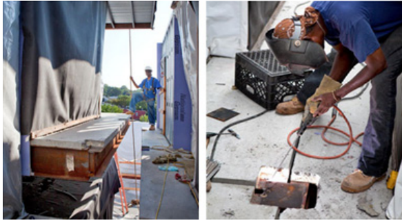
Fig. 6. Connection system of Capsys Corporation
