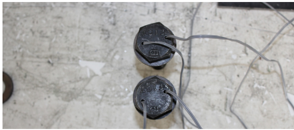
Fig. 8. Strain gauge install on H.T.B
