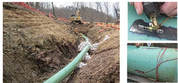
Fig. 1. VW-strain gagues installed along the bottom of slopes.
