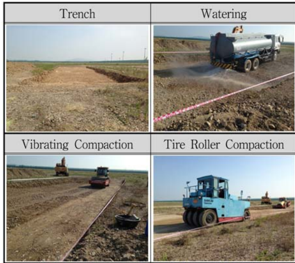
Fig. 4. Procedure of field compaction.
