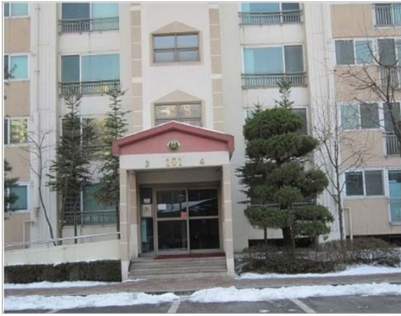
Fig. 1 Front view of Hyundai Jookjeon Hometown apartment.
