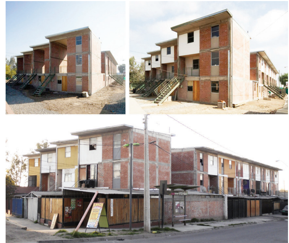
Figure 8. (above) Initial incremental phases of Elemental Lo Espejo, Elemental, (2006 and 2007), Source: http://divisare.com/projects/280780 -ELEMENTAL-Alejandro-Aravena-Lo-Espejo (below) of Elemental Lo Espejo houses after customazation, (2015), Source: by author
