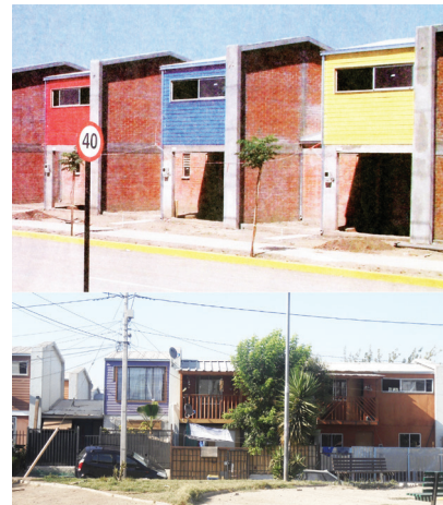
Figure 9. (above) Las Higuera before extension of houses, (2006), Source: Pamela Suarez, "La Salida de la Toma de Peñalolén," Institute of Ecological Neighborhood. (below) Las Higuera after extension of houses, (2015), Source: by autor
