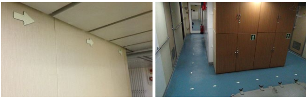
(a) Exit Guidance attached at wall (b) Exit Guidance attached at Floor
