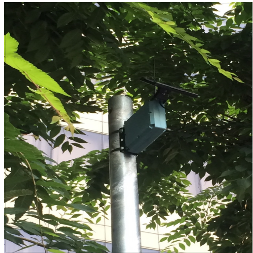
〈Fig. 5〉 Shady location Field collection device installed
