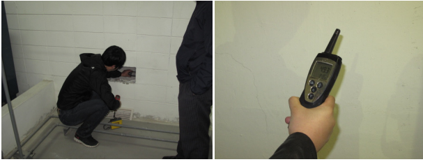
Fig. 1. Temperature-humidity measurement in underground parking lots(Testo 625)
