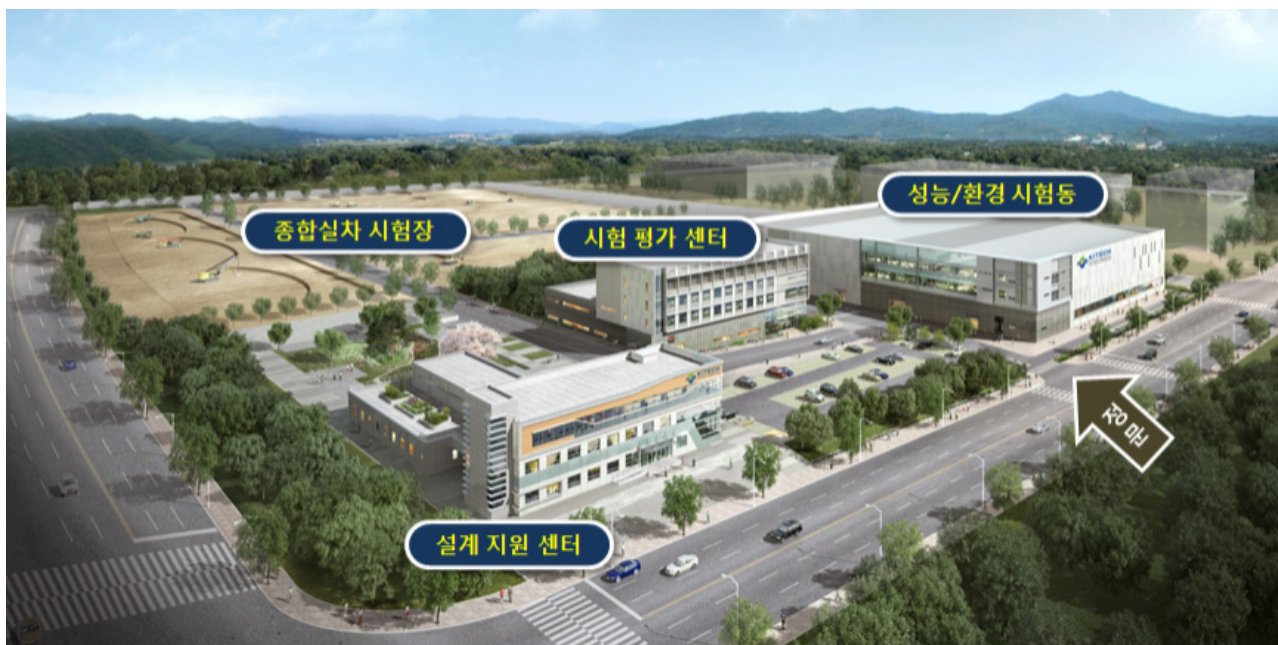
Fig. 1 Construction summary of Construction Equipment Technology Center
