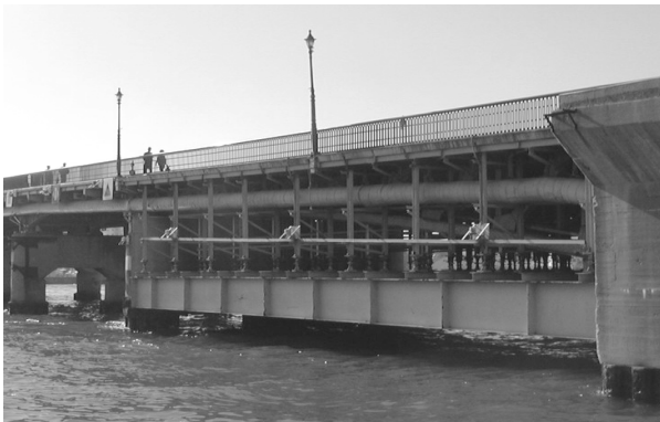
Photo 1 Yeongdo bascule bridge in 2002
