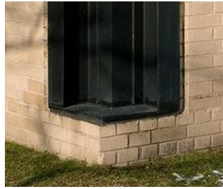
<그림 2> Mies van der Rohe, Alumni Memorial Hall at IIT, detail of corner beams and bricks
