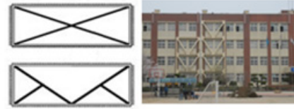
Fig. 3. Construction case of steel brace
