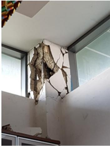
Fig. 1. Short-column shear failure observed in 912 Gyeongju earthquake
