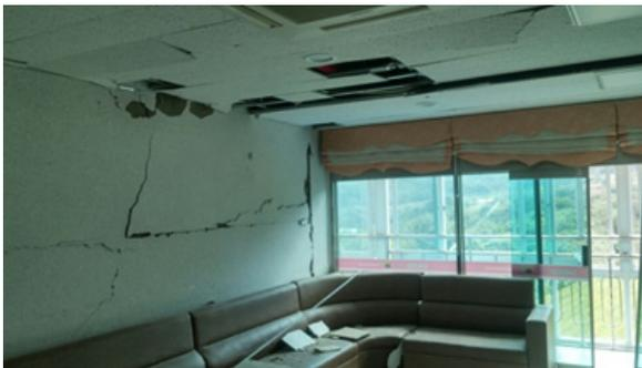
Fig. 2. Cracking of infilled wall and ceiling failure observed in 912 Gyeongju earthquake
