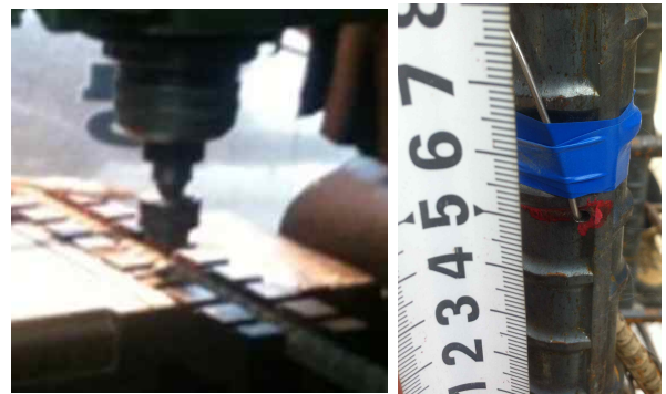
Figure 6. Installation of sensor
