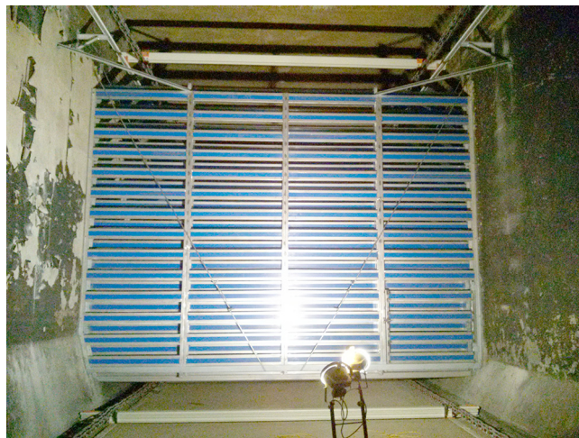
(b) Picture of double rectification wall in 2nd sedimentation tank
