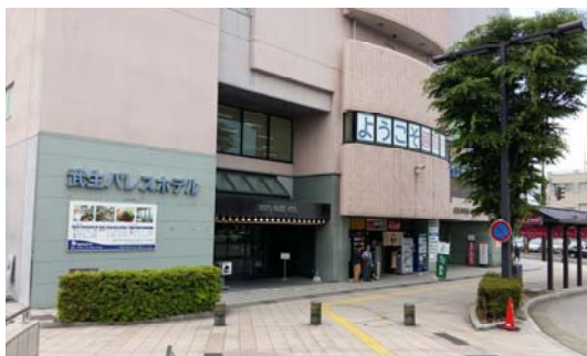
Fig. 1. Private building where 5 administration department such as commercial/tourism promotion section are positioned.
