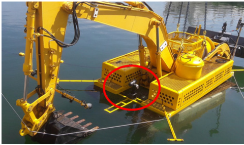
Fig. 8. Installed sonar at underwater equipment for rubble mound leveling
