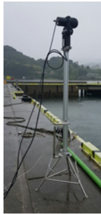
Fig. 2. Sonar and pantilt installed zig
