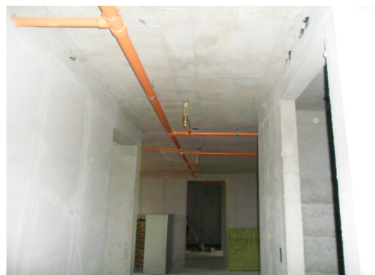
Fig. 5. Construction case of CPVC pipe
