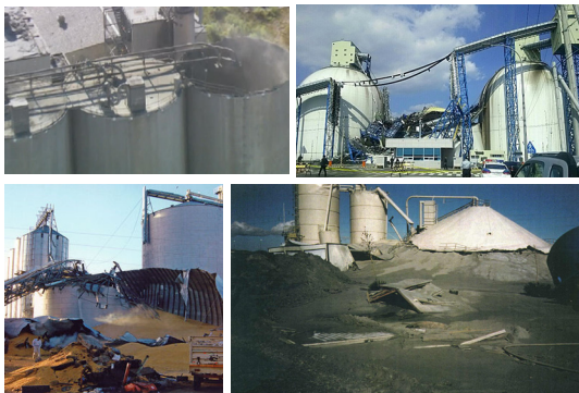
Fig. 2. Examples of silo collapse
