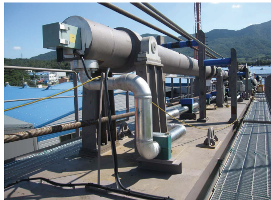
Fig. 14 Installation of System for 50 ton desk crane
