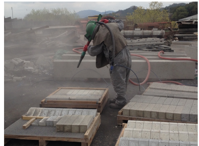
(a) Shot blasting
