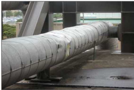
Fig. 1. Pictures of damaged fixed-insulation.
