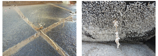
(e) Waterproofing sheet surface observation (f) Roots penetration observation
