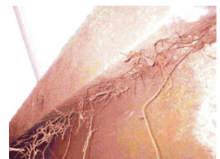
(b) Leakage caused by plant roots
