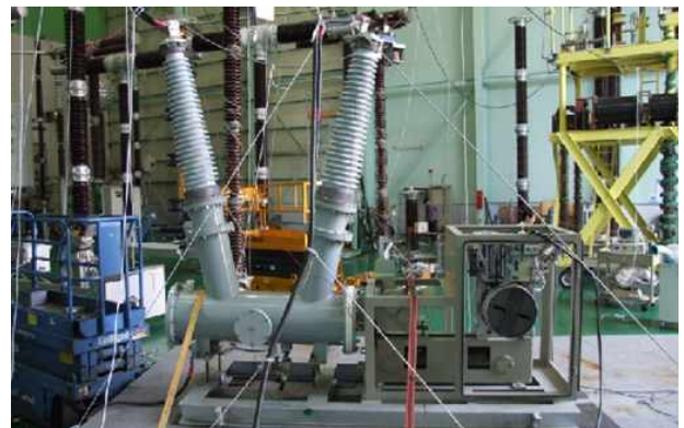
Fig. 7. Installation of a 145kV self-blast gas CB in the testing room.
