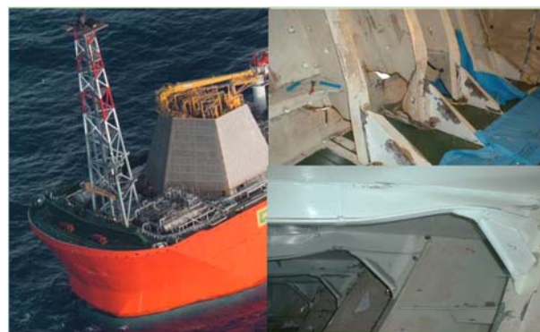
Fig. 2 Damaged shape of the Schiehallion FPSO
