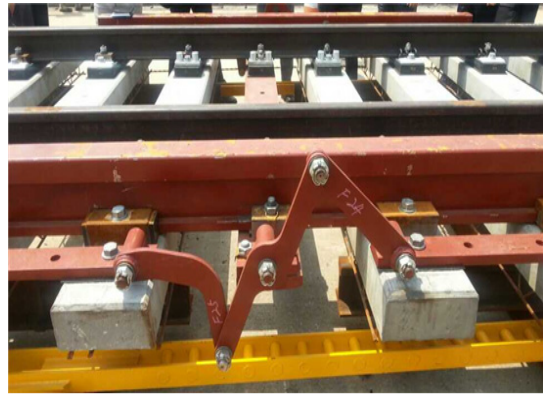
Fig. 1 A special device to support the rail at the center of a large sleeper span
