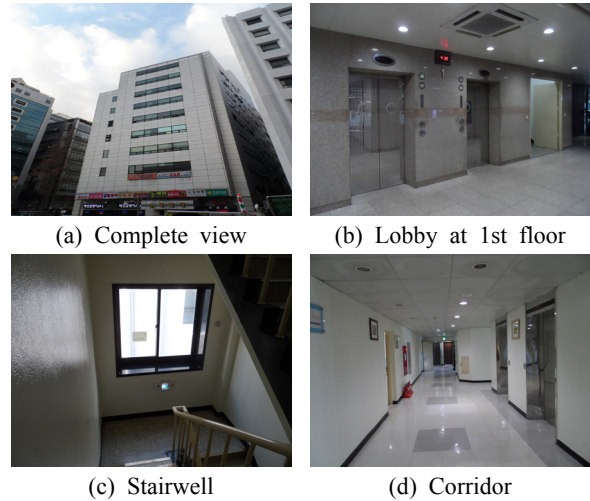
Fig. 2 Photograph of building structure.
