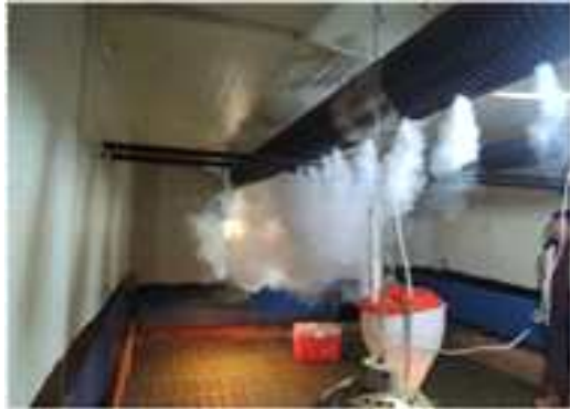
Fig. 3. Picture of air flow from duct hole installed in pig house.
