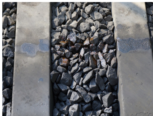
Fig. 6. Railroad site to which in-situ Fenton oxidation was applied.
