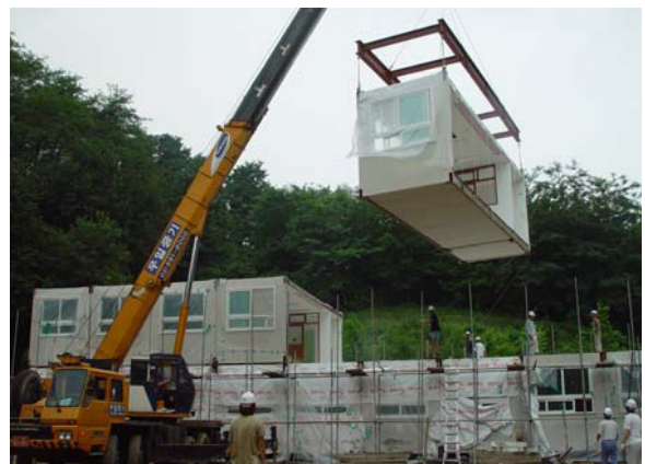
Figure 1 Modular school (Singi elementary school)
