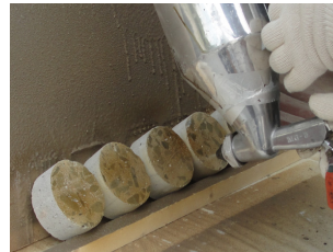
(a) Application of the coating agent
