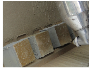
(a) Application of the coating agent
