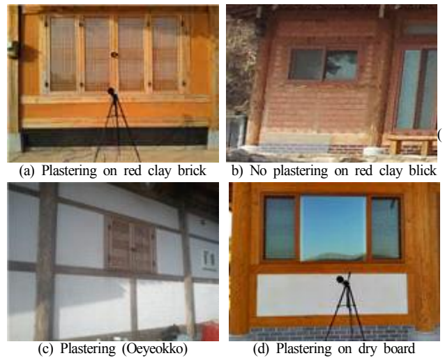
Fig 2. Scene of plastering on main wall material
