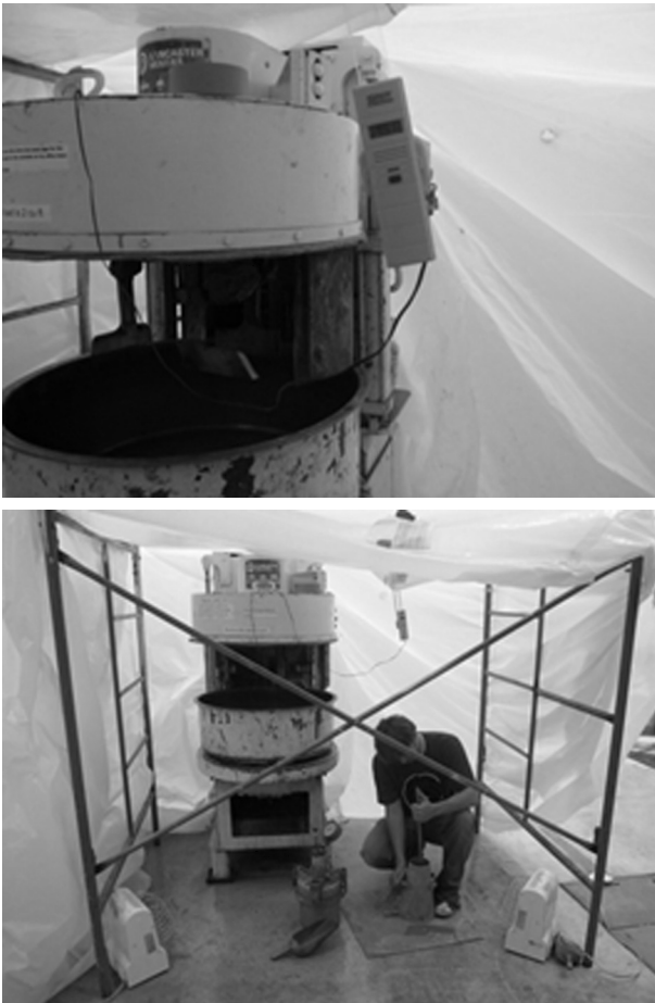
Fig. 1. Testing set-up used for the high temperature, extending mixing procedure: pan mixer and air temperature sensor control system (up), enclosed testing area around mixture showing space heaters and fresh concrete test equipment (down).
