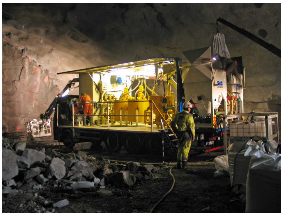
Fig. 4. Modern grouting rig for high pressure pre-grouting
