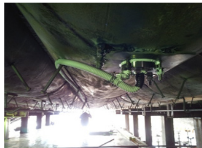
(b) Installation of sensor ②
