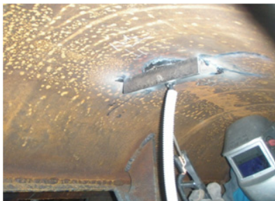
(a) Installation of sensor ①
