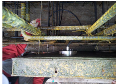
(b) Sensor④ on formwork
