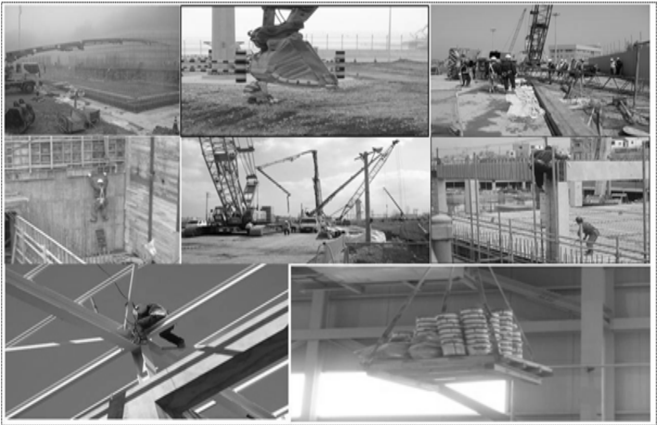
[Figure 2.2] The work type of plant construction site
