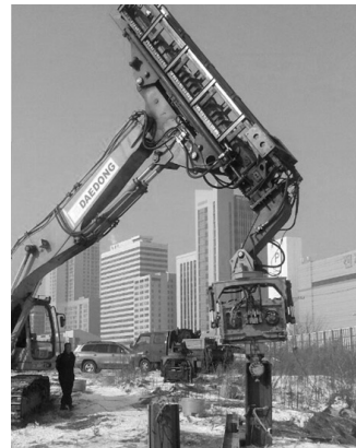
(b) leader-mounted vibratory-machine system
