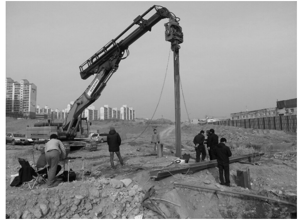
(b) Hydraulic type & Variable amplitude type
