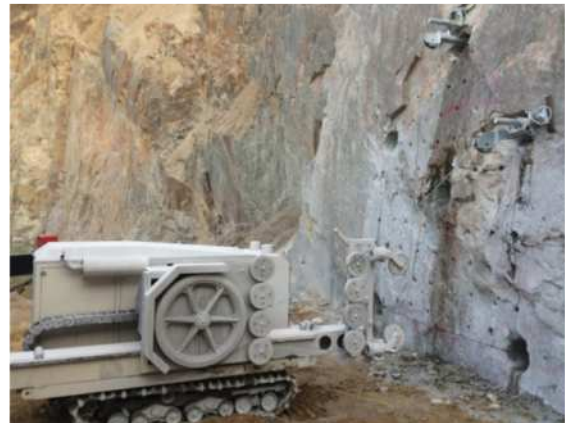
Fig. 10 Wire saw cutting test in field
