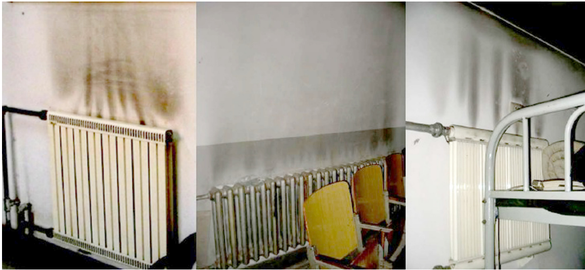
Fig. 1. Examples of the particle deposition on walls above radiators.
