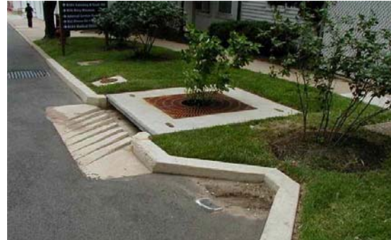
Fig. 3. Illustration of filtering system in treebox filter.
