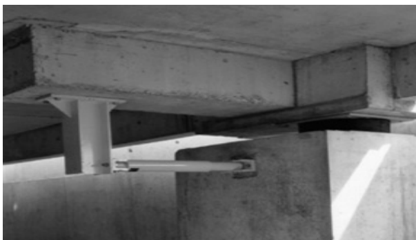
(b) Isolator Protection by Damper Devices
