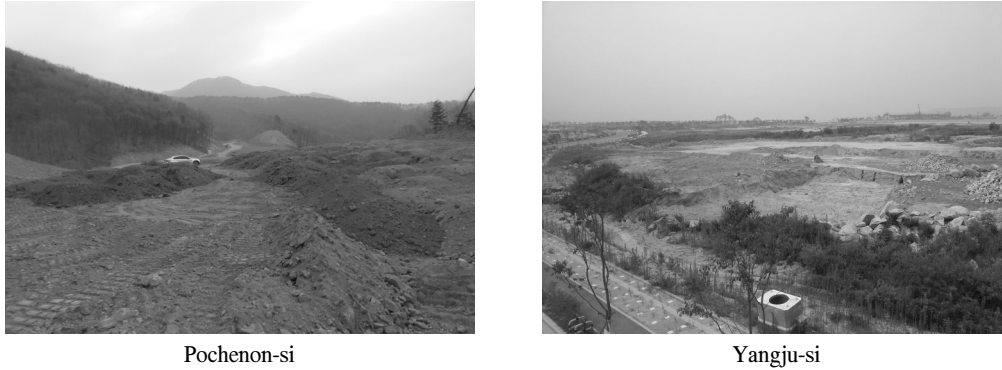
Figure 1. Construction site view.
