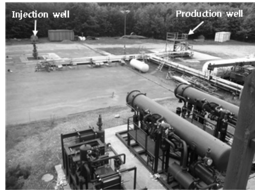
Fig. 3. Groß Schönebeck EGS research site in northern Berlin (picture taken in May, 2015). Production well is in the upper left and injection well head is in the upper right. The distance between injection and production well is 28 m on the surface and 475 m at the final depth. Binary geothermal power plant with the capacity of 1.1 MW is also in place. The site is located far from the residential area and the total area of the site is around 6,000 m 2
