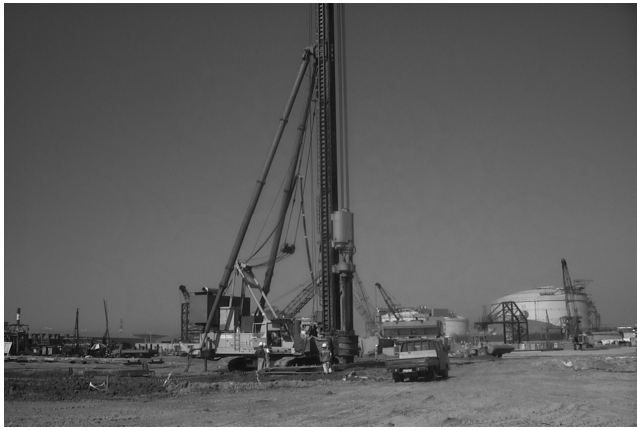
Fig. 11 SMW mixing test for soil excavation in site
