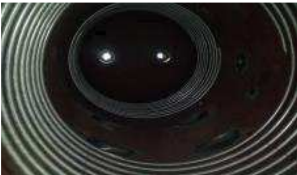
Fig. 7 Circulation of refrigerant piping
