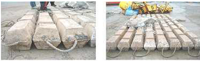
(a) Rope integrated FCM in Singapore
