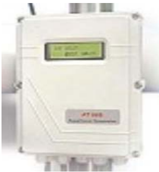
Fig. 7 GE AT868 controller
