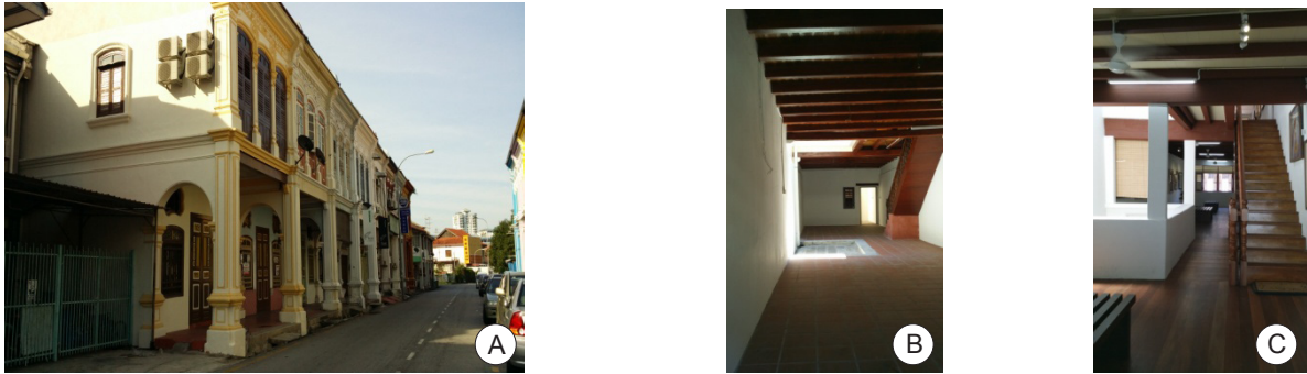
Figure 3. (A) English influence shop house arcade. (B) Inner air well (ground floor). (C) Inner air well (1st floor) (photo by author, 2014 in George Town, Penang).
