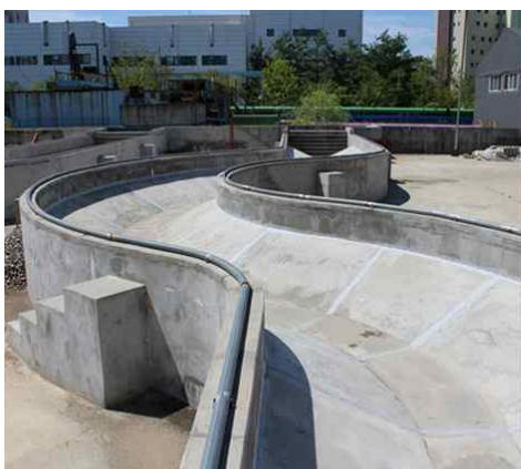
(a) The meandering channel in Korea Institute of Civil Engineering and Building Technology
